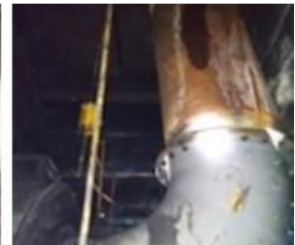
poor sealing
