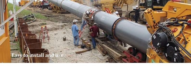
It can be installed by flange, quick connector and direct welding.
